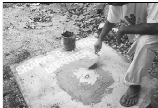
Figure E2. Concrete Vault Being Sealed
